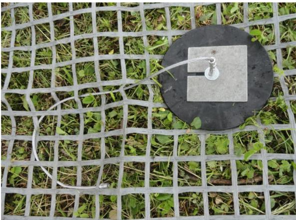
A photograph showing the cable anchor installed on the metal grid. The anchor is now secured to the grid. The grid is made of galvanized steel and is set on a concrete base. The background shows green grass and a black circular object.                                                                 | <p>Enfiler le reste du câble de l'ancrage sous la grille à hautes performances S&amp;P.</p>                                                                                                |
